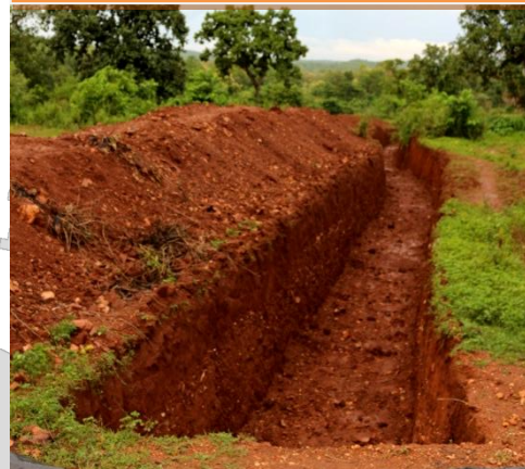
Figure 24 : Elephant Proof Trench at interstate border
