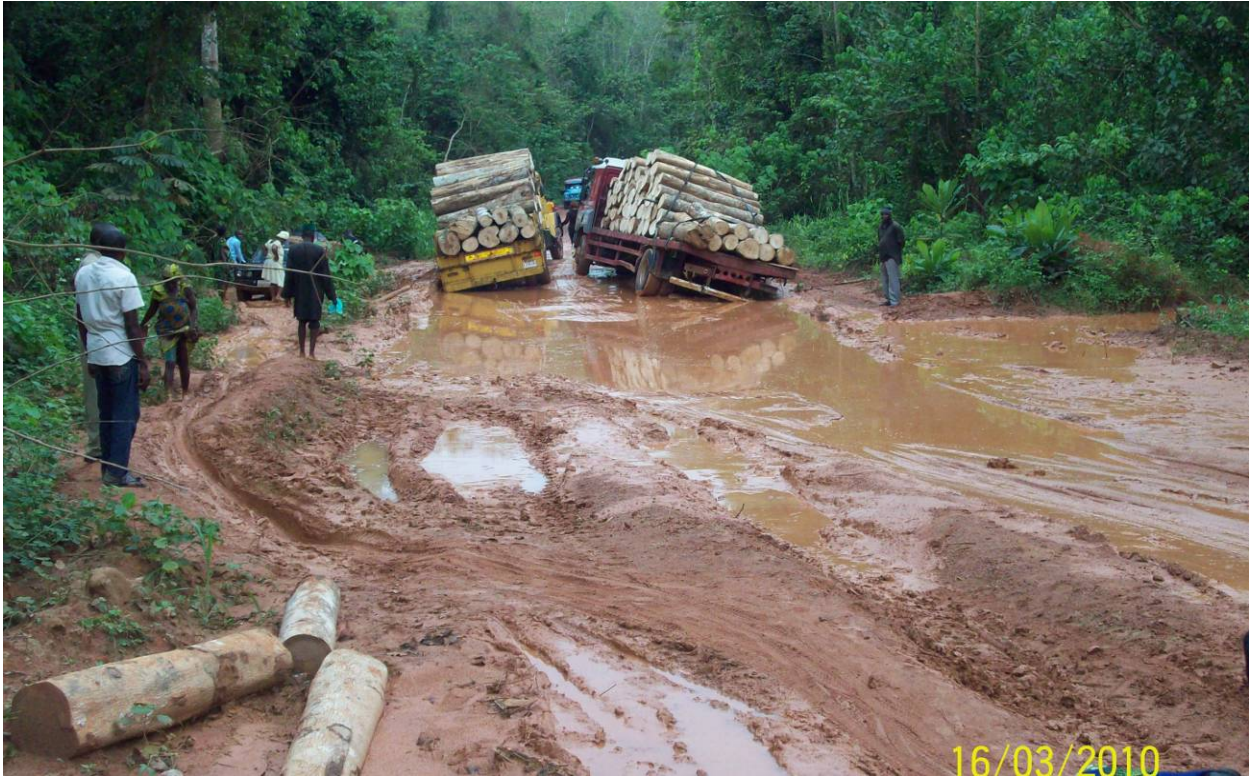
Poor Quality of the Road Network in Omo Forest Reserve
